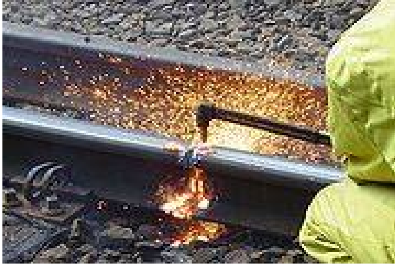
Figure6.8: Manual Gas Cutting
